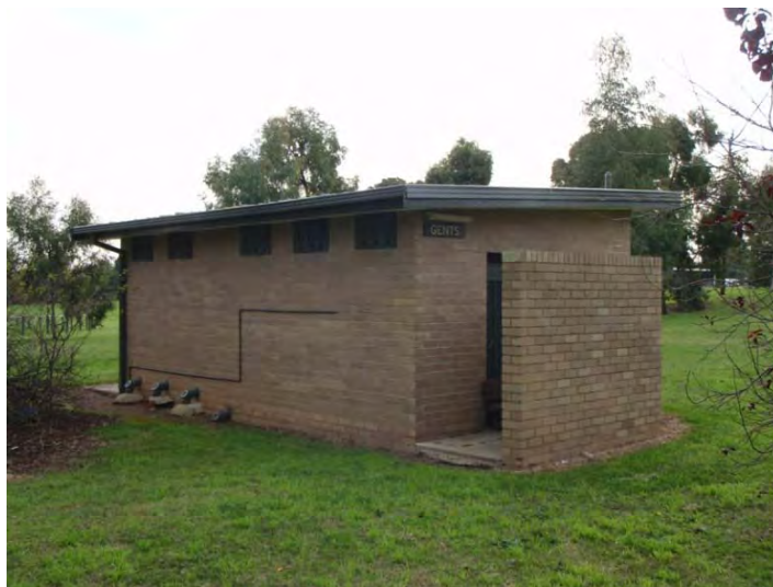
Figure 17: Southern Toilet Block
