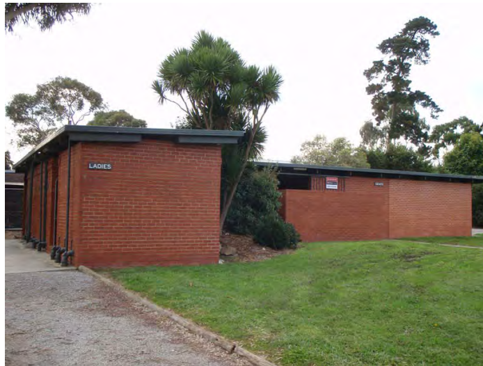
Figure 7: Central Toilet Block
