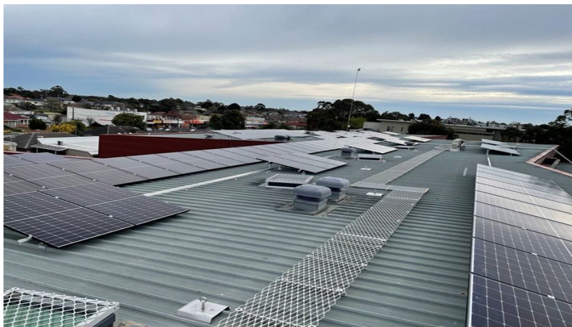
Solar at Clayton Community Centre
