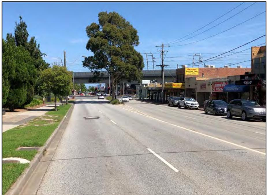
**Carinish Road** is a Council managed Collector Road, that essentially runs in a northwest – southeast alignment. The road has a carriageway width of approximately 12.5 metres accommodating one traffic lane in each direction along with kerbside parallel parking provided on one side of the road. Carinish Road has a posted speed limit of 50 km/hr. Footpaths are provided along both sides of Carinish Road.
