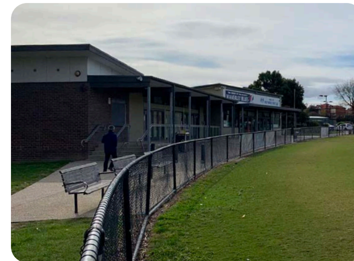
Football/cricket pavilion viewed from the south.
