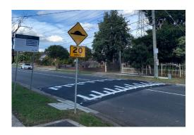
The road humps would be full width and lower in height. The modified flat topped road hump is lower than a standard hump (75mm high instead of 100mm). It provides a smoother drive and reduces noise, while still addressing speed concerns.
