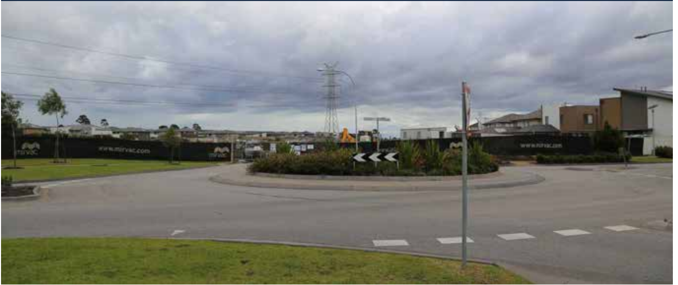
View of existing central tower from southern end of Queensberry Circuit
