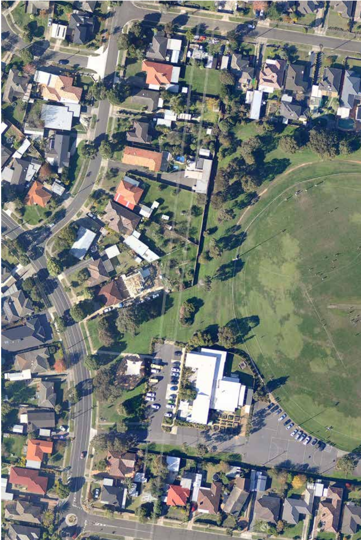
Transmission lines over rear yards, open space and car park Mackie Road and Redfern Crescent, Mulgrave
