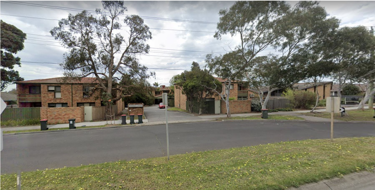
Picture 6 1498-1502 North Road, directly East of the subject site
