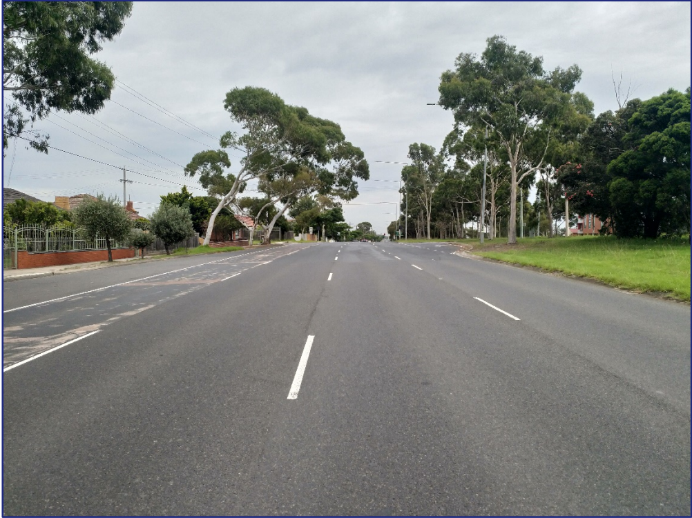
Figure 5: North Road – view west
