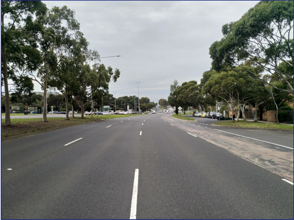
Figure 4: North Road – view east
