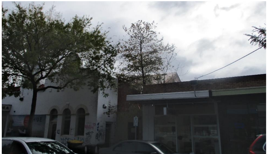
Photo 2-5: Buildings to the east of the subject site
