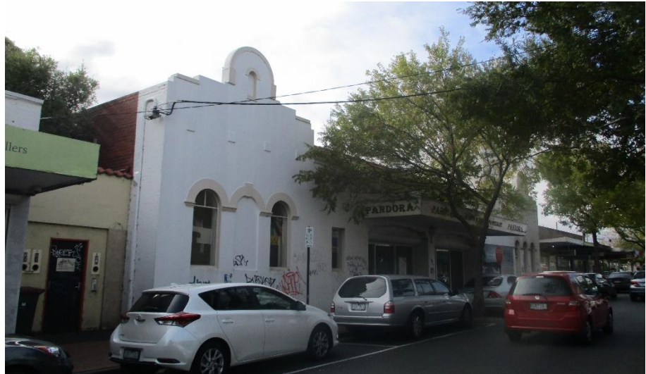
Photo of existing street wall
