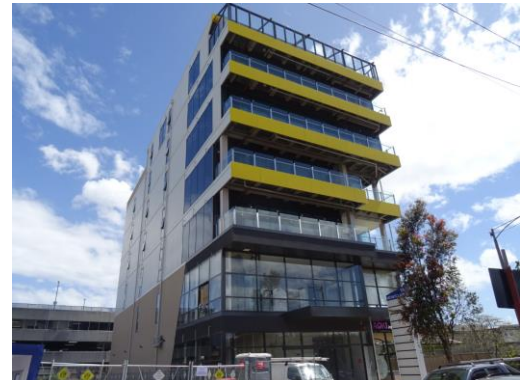
East – 7 storey commercial building at 52 Montclair Avenue
