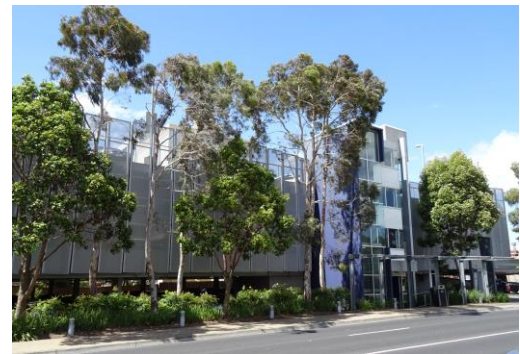
South - Bogong Avenue 3 storey car park (looking north)
