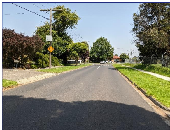
Figure 8: Beryl Avenue - view west
