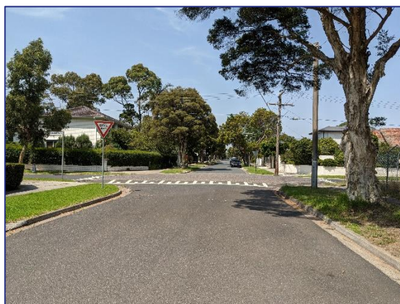
Figure 10: Bakers Road - view south
