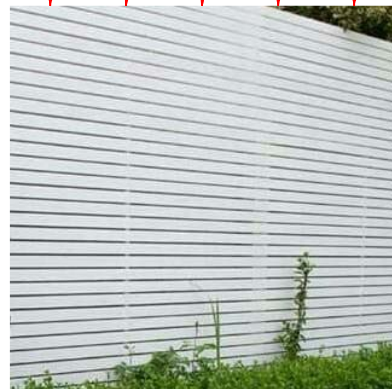
FT03 FENCE TYPE 03 - METAL SLAT FENCE PAINT FINISH: OFF WHITE OR SIMILAR
