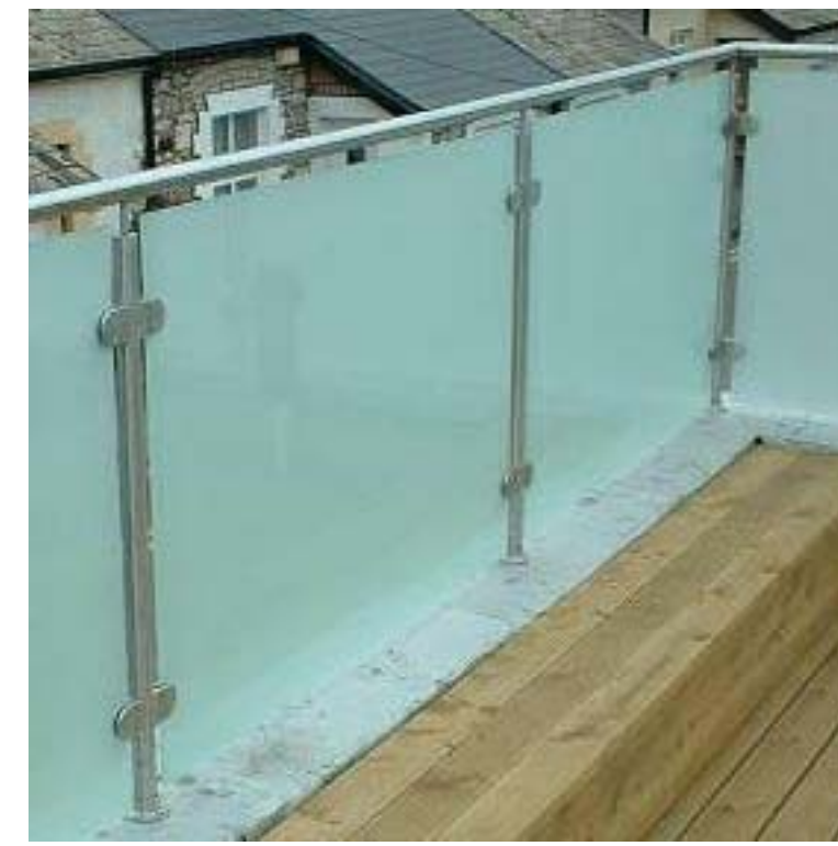
BT02 BALUSTRADE TYPE 02 GLASS INFILL: OBSCURE BALUSTRADE & HANDRAIL: STAINLESS STEEL OR SIMILAR
