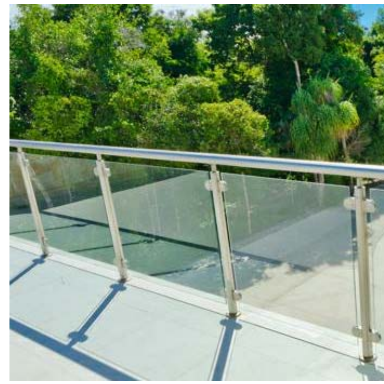
BT01 BALUSTRADE TYPE 01 GLASS INFILL: CLEAR BALUSTRADE & HANDRAIL: STAINLESS STEEL OR SIMILAR
