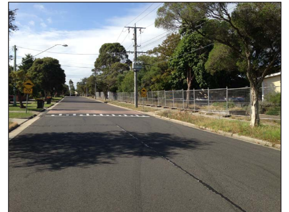
Figure 2.3: View of Browns Road, Facing North in the Vicinity of the Site
