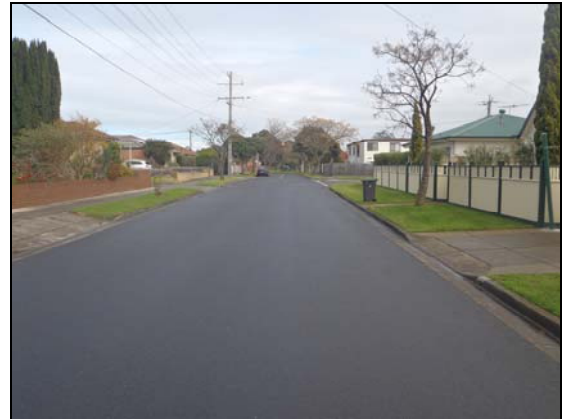
Figure 9: Coombs Avenue Looking West
