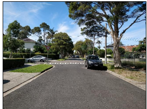
Figure 12: Bakers Road – view south
