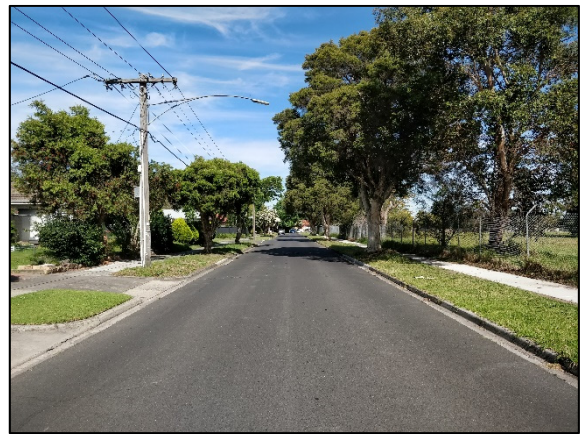
Figure 10: Beryl Avenue – view west
