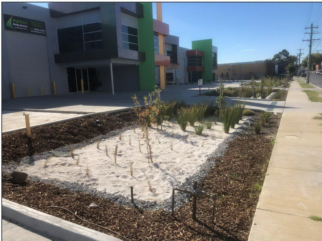
Figure 12: Example of Raingarden in An Industrial Development
