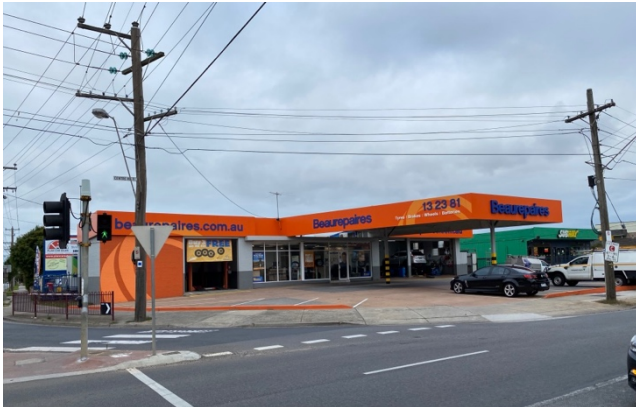
Figure 11: Photograph of Centre Road, opposite the Subject Site to the south
