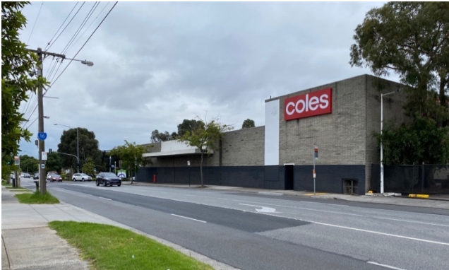
Figure 12: Photograph of rear of Coles Supermarket, Centre Road frontage, immediately to the west of the Subject Site.
