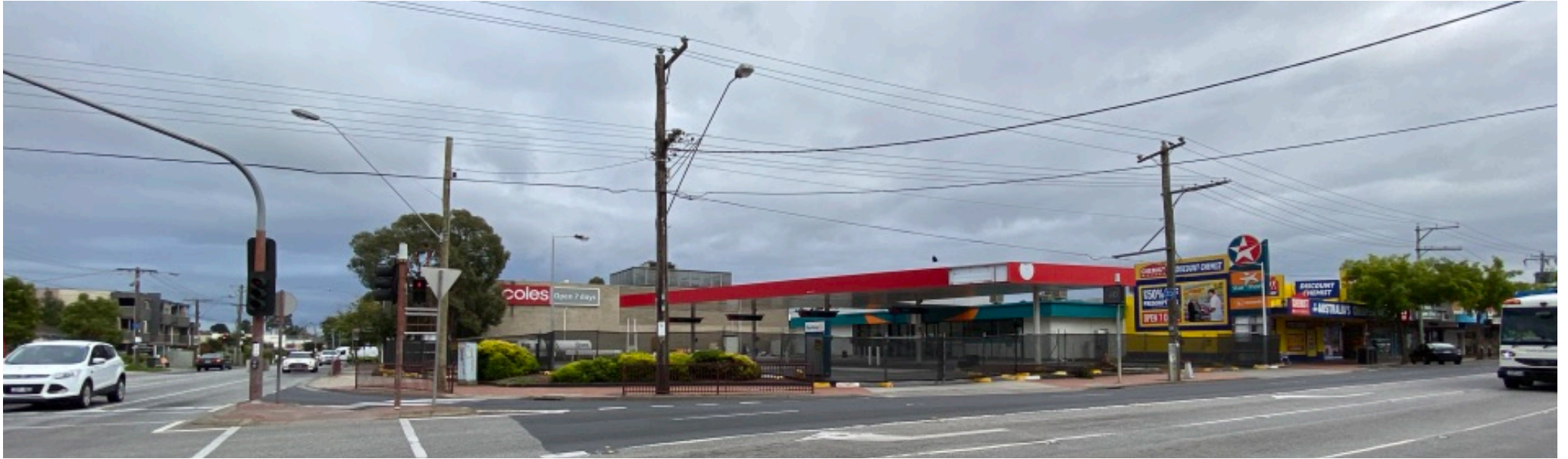
Figure 6: Subject site – Clayton Road Frontage (note: photo taken pre-demolition and remediation)
