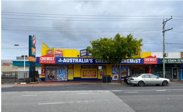
Figure 7: Photograph of 405-407 Clayton Road
