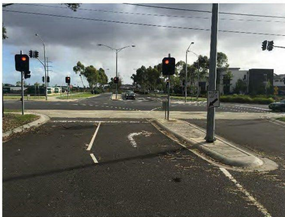
Figure 12: Jacksons Road / Gate Seven Drive – Eastern Approach
