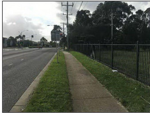
Figure 5: Jacksons Road – View North
