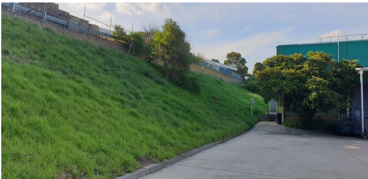
Figure 4. Level Change 636 Wellington Road (left of shot) and 1 Jacksons Road (right of shot)
