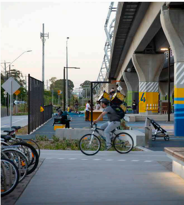
Image 19. Upgraded shared path infrastructure
