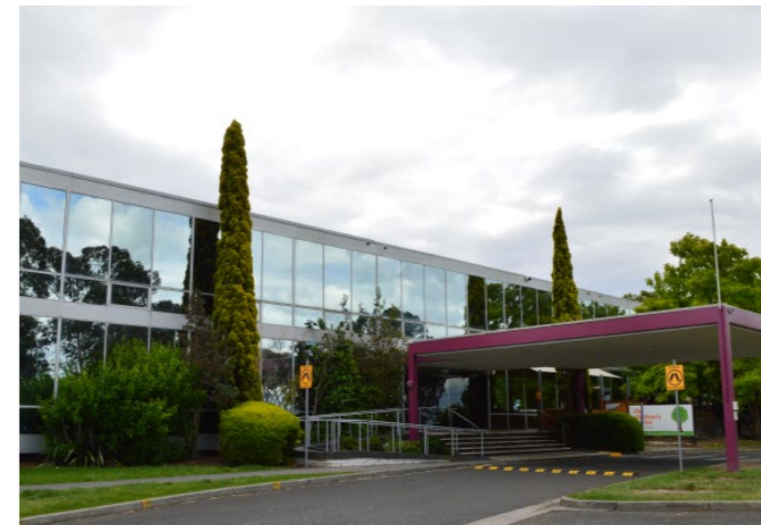
2) Double-storey office building
