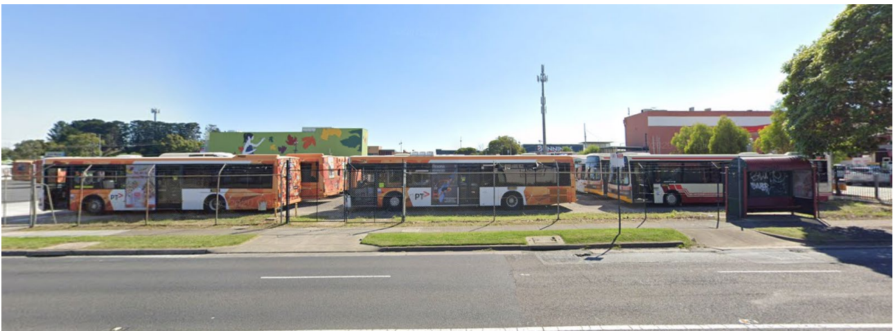
Picture 9 Ventura Oakleigh Bus Depot Centre Road
