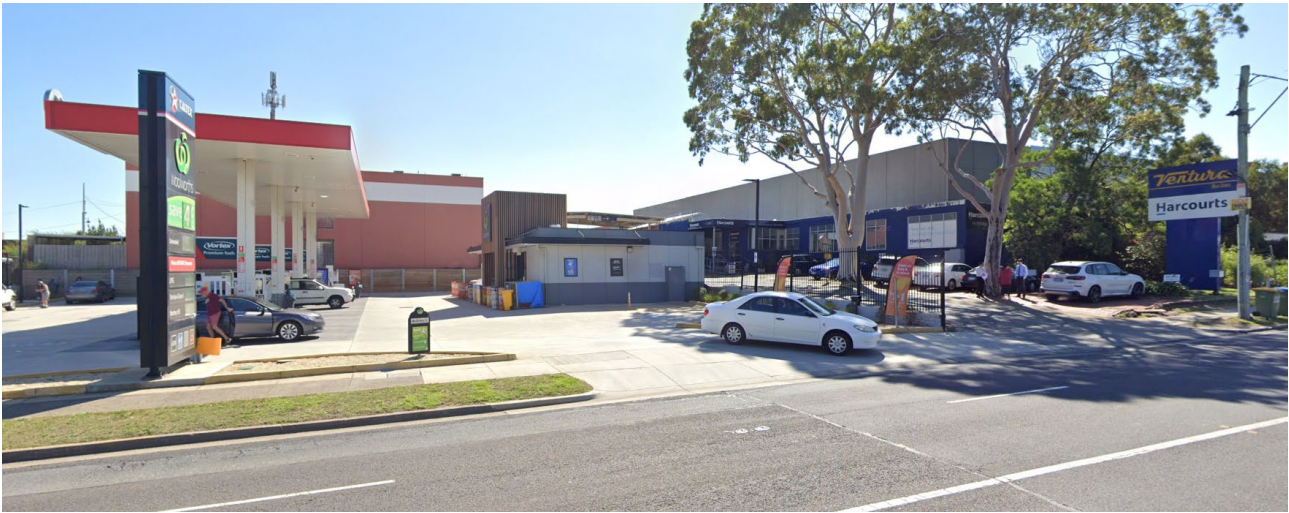
Picture 8 Service Station No.1033 Centre Road, Oakleigh South
