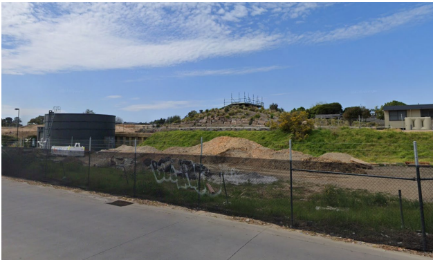
Picture 5 BMX Track from Link Ave
