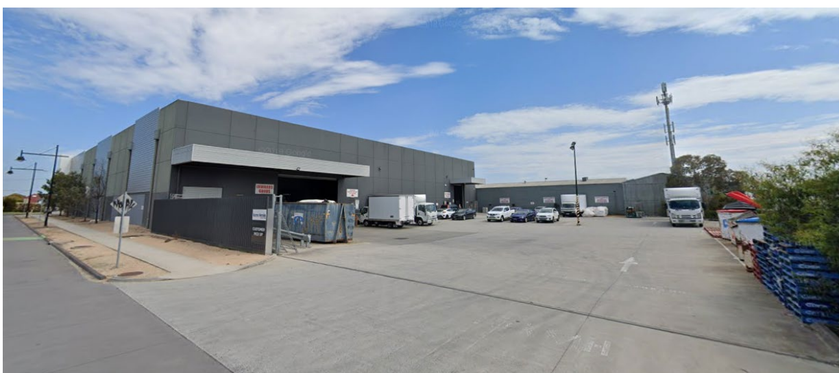
Picture 2 Existing subject site conditions (from Links Ave)
