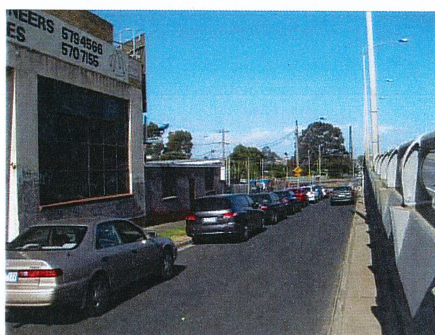
North Road off-ramp
