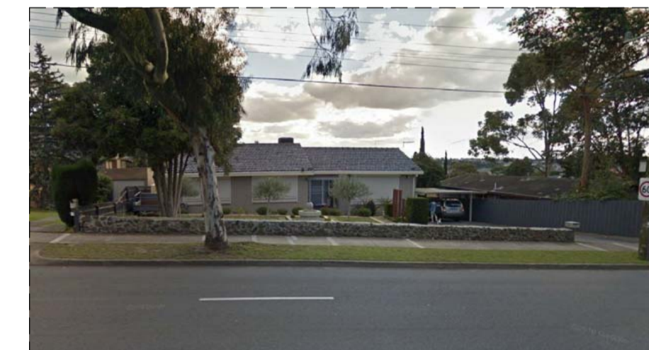
No. 87 Huntingdale Road (Subject Site) Single-storey brick veneer with pitched roof
