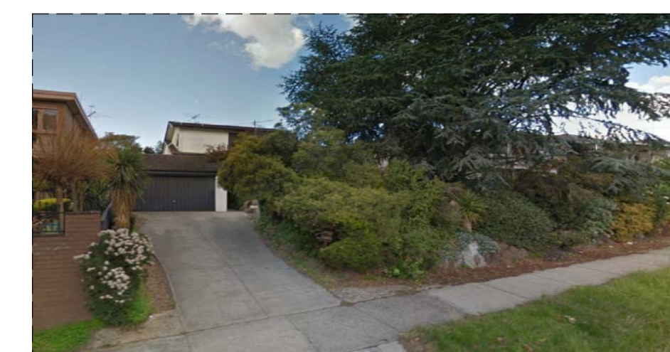
No. 130 Huntingdale Road Double-storey rendered brick with pitched roof
