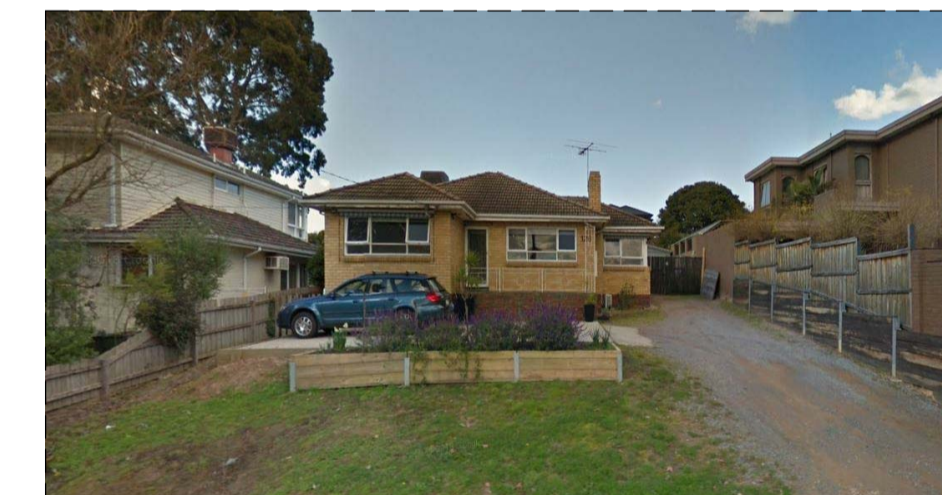
No. 126 Huntingdale Road (Subject Site) Double-storey timber with pitched roof
