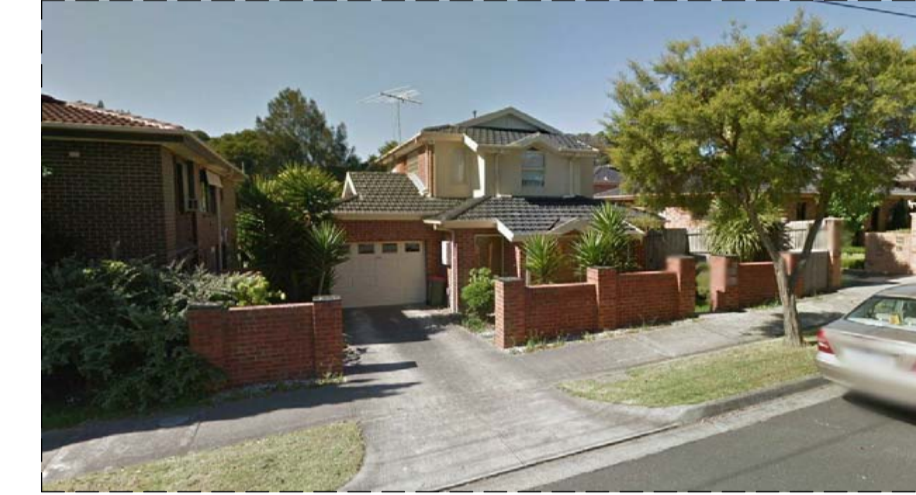
No. 2/120 Huntingdale Road Double-storey brick veneer with pitched roof
