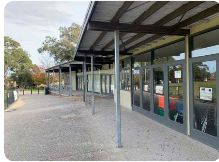
Pavilion with concrete apron
