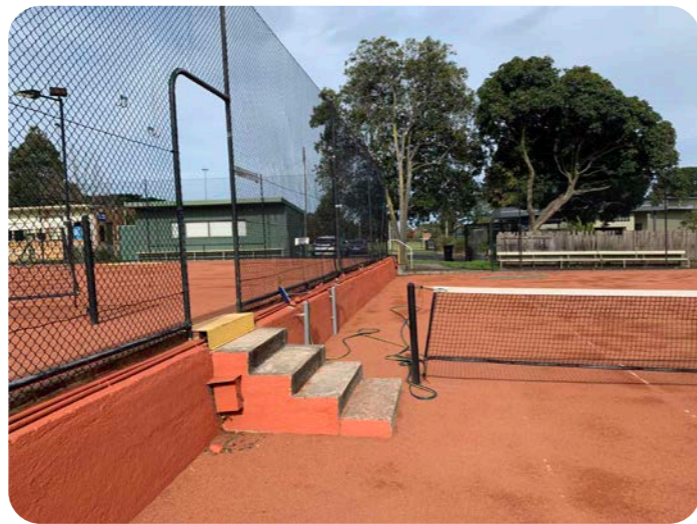
Western-most tennis court with retaining wall
